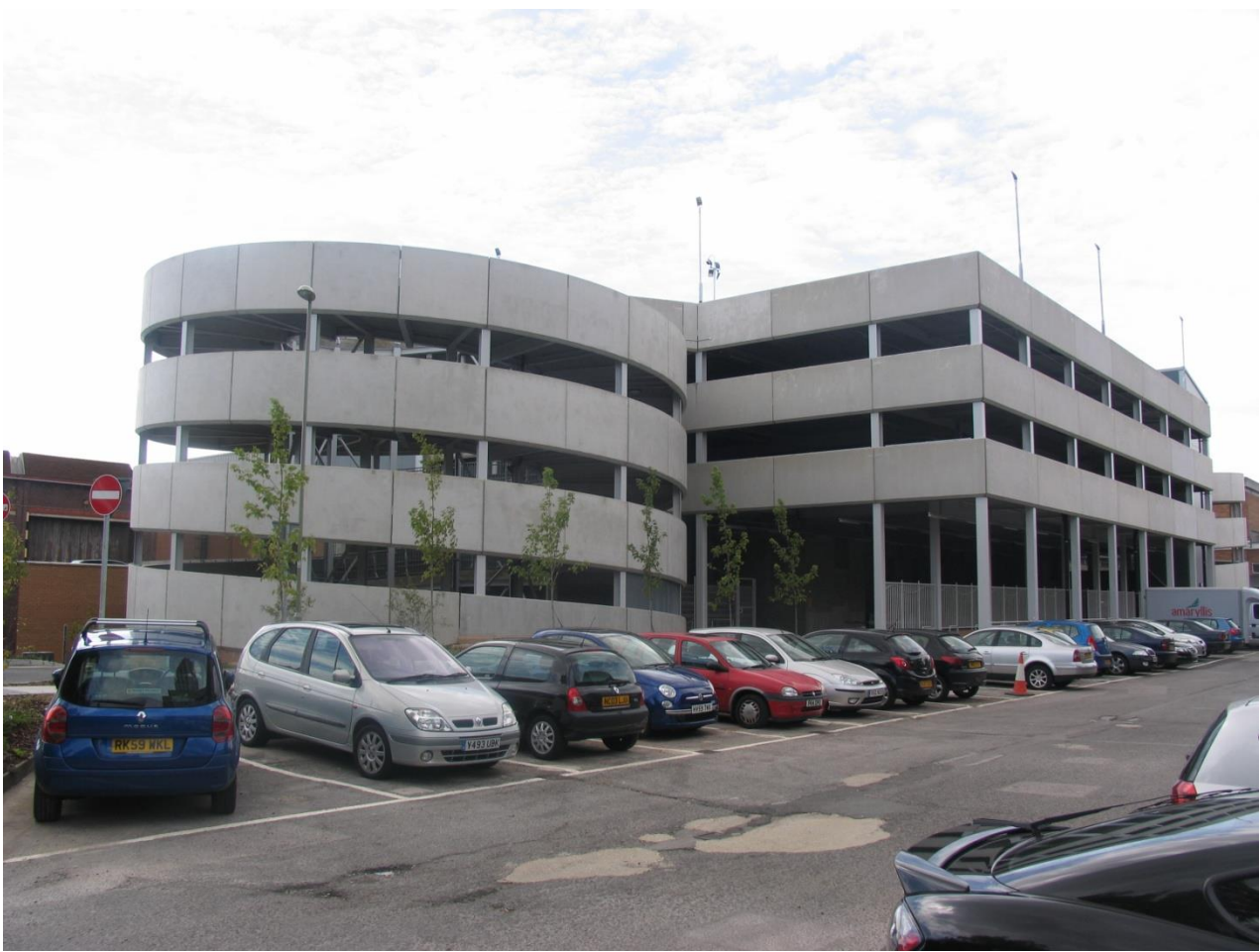
Fareham Shopping Centre Multi Storey car park
